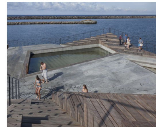
Figure 98: White Architects. Hasle Harbour Bath. 2013. Photograph by Signe Find Larsen. ArchDaily.
