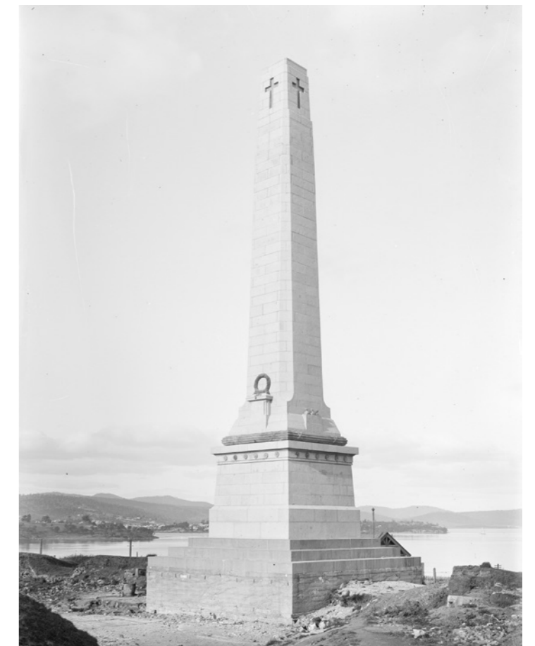
Figure 37: The Cenotaph during construction, 1925. (TA, NS1013/1/155, Photograph - Cenotaph nearing completion.)
