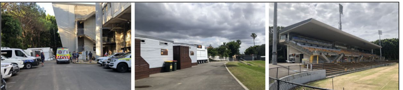
Figure 4 | On-site parking (left), demountable bathrooms and bar above the hill (middle) and Western Grandstand (right) (Source: EIS)
